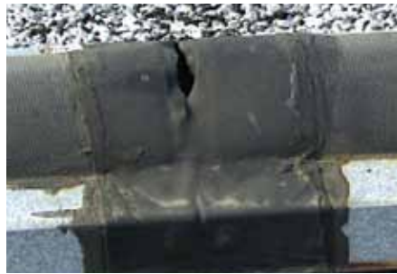
Splice failure on competitor's product
